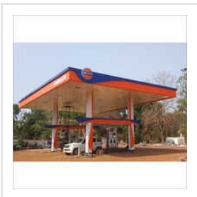
Indian Oil Petrol Pump Canopy
