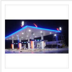
Hindustan Petroleum Petrol Pump Canopy
