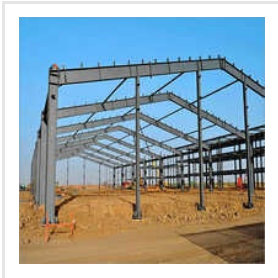
Industrial Iron Structure Canopy
